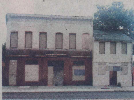
BALTIMORE DEVELOPMENT CORP. PHOTO The Sphinx Club closed in 1992 and is now city-owned property.
